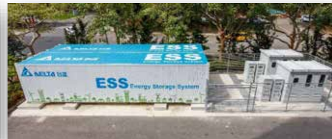
500kW/3MWh Hsinchu, Taiwan Demand response, power backup, peak shaving, frequency regulation, load shifting
